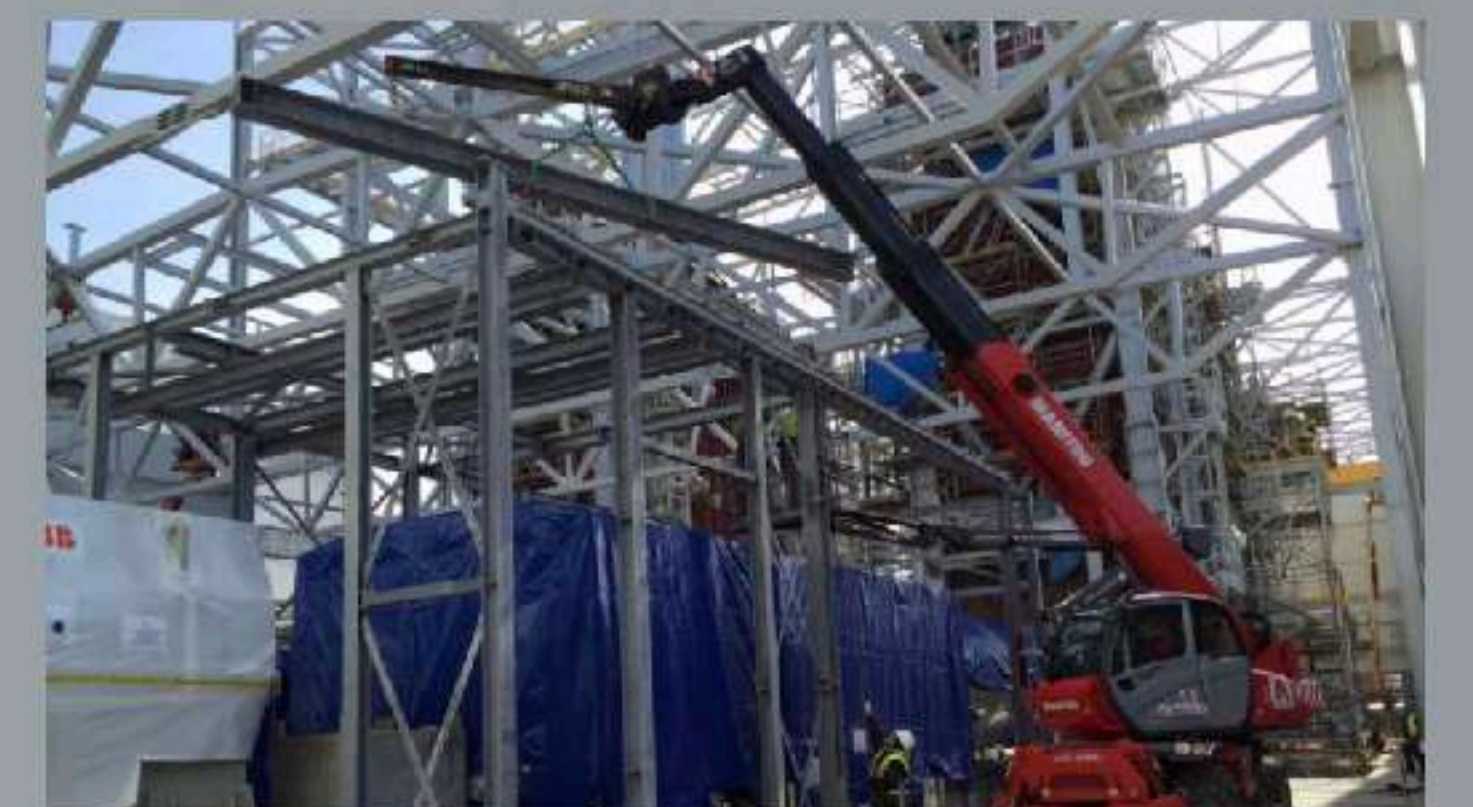
Steel structure and insulation panels
