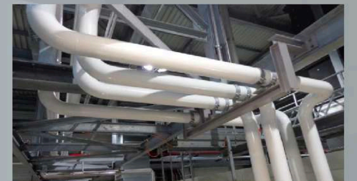
Piping fabrication and installation
